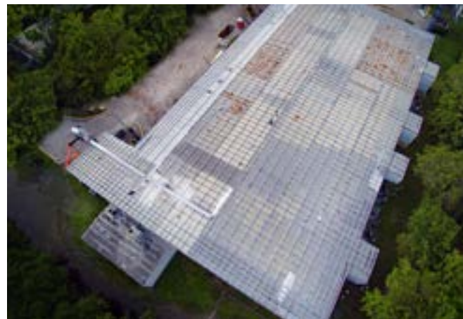
Aerial view of roof grid. PHOTO COURTESY OF MCELROY METAL
