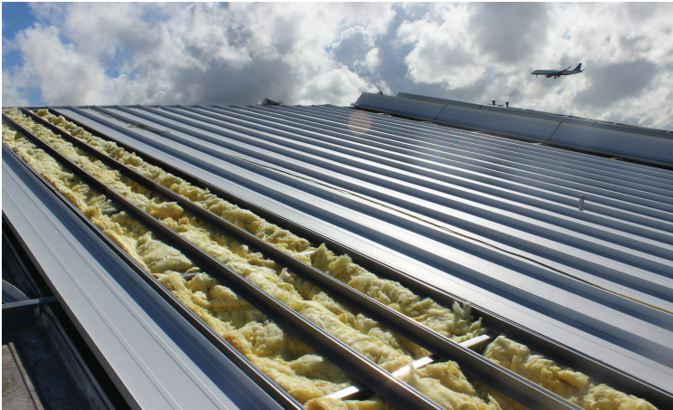
Figure 2: Metal roof installation in progress over an existing metal roof
