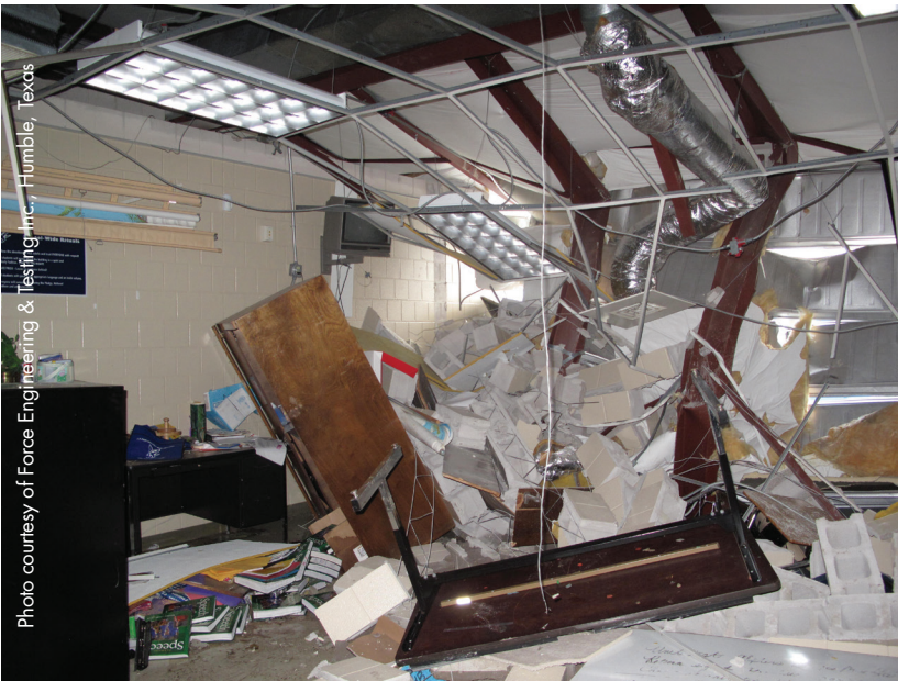
Figure 7: The interior of a building following roof structure failure
